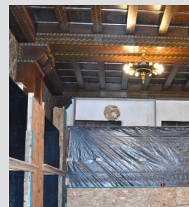
With the original wall covering gone, above, HVAC contractors removed the 1960's duct work and exposed the original vent holes. Right, they then installed the new ductwork in the original locations. Below, plasterers repaired the walls, adding plaster where needed. The conservator then worked to reinstall the linen wall covering and fill in missing sections.
