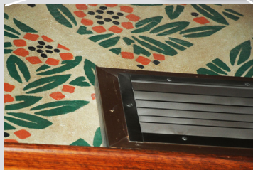
Above and right, the linear vent was cut into the wall and through the hand-stenciled linen wall covering.
