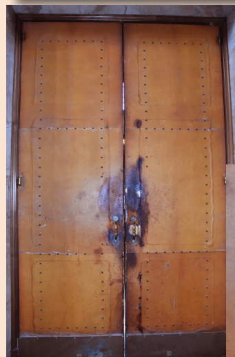
Left, the Library door's leather covering was torn and damaged from years of use. Below, in addition to missing leather, some of the decorative studs holding the leather in place are missing.
