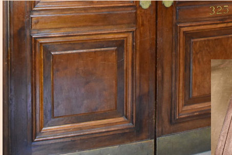
Left, the Library doors show years of use; the doors were scratched and soiled. Below, once hardware was removed staff cleaned the grime and refinished the scratches.
