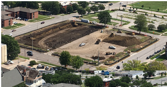
July of 2018 wellfield site preparation began with the removal of the parking lot surface, the remaining structures, and the rerouting of all on site utilities.
