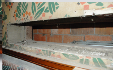
Above, the ventilation system added to the courtroom in the 1960's was oversized and not compatible with the room's historic character.
