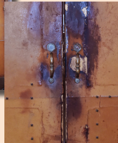
Left, the Library door's leather covering was torn and damaged from years of use. Below, in addition to missing leather, some of the decorative studs holding the leather in place are missing.
