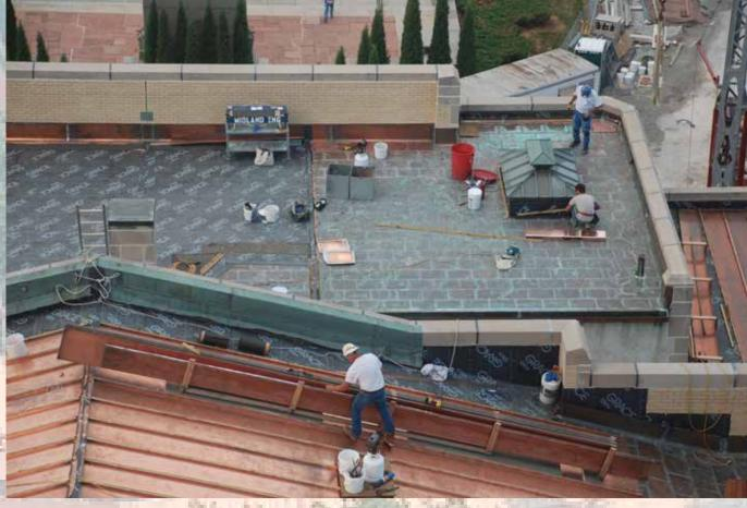
A new copper batten and flat lock roof system was applied over a waterproof membrane and insulation. Insulation was added where none existed originally. Replacing flat lock panels with a batten system decreases the number of seams reducing the potential for leaks. Wall flashing was extended to reduce ice dams causing leaks.
