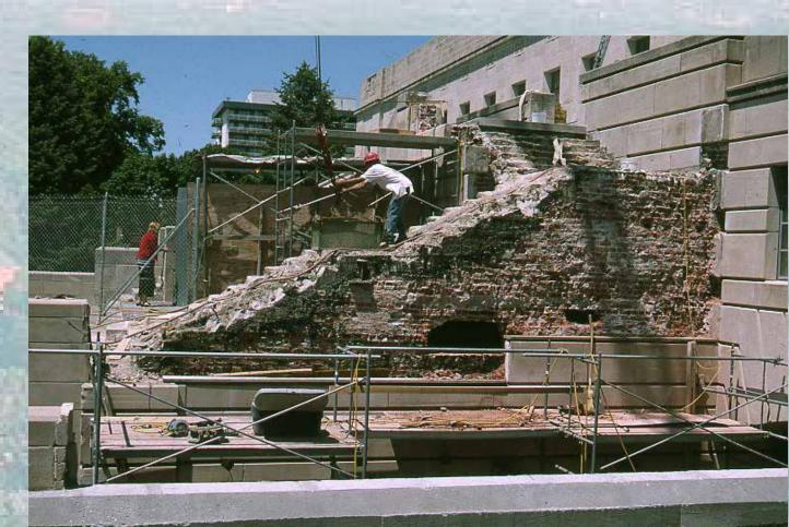
Restoration of all four entrances required removing and storing the limestone façade and granite stair treads, then demolition of the red clay brick core down to the foundation. The interior core was rebuilt using poured concrete
