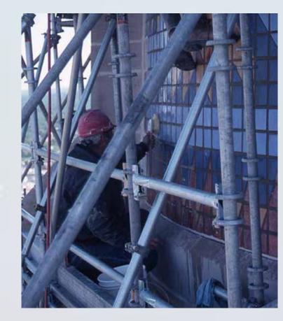
Inspection of the gold tile dome and tile Thunderbird mosaics revealed they were in good condition. Restoration involved cleaning with soapy water and adding grout where necessary. The limestone exterior was cleaned using a biocide followed by a low pressure air abrasive process.
