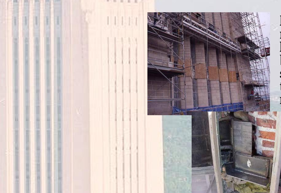
Relieving stresses in the tower required the removal of limestone veneer at each floor level. Contractors then removed the brick backing to reveal the tower's structural steel frame. Shelf supports were attached to the floor beams and the limestone veneer reapplied to rest on the supports. The
