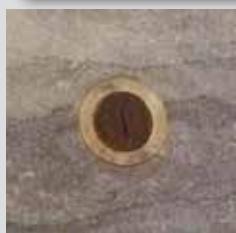
Above, it took OCC's mason Dan Kratky 20 minutes to drill the hole that houses the floor port, left, which will allow easy access to electricity and data beneath the bailiff's desk.
