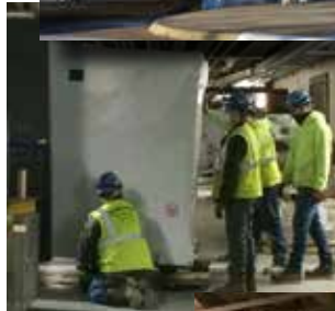
Right, the units are joined and ducts attached to move the conditioned air throughout the Capitol.
