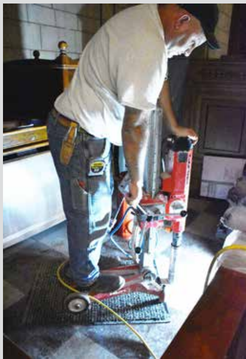
Above, it took OCC's mason Dan Kratky 20 minutes to drill the hole that houses the floor port, left, which will allow easy access to electricity and data beneath the bailiff's desk.
