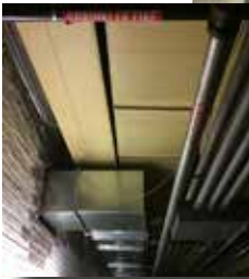
Right, the units are joined and ducts attached to move the conditioned air throughout the Capitol.
