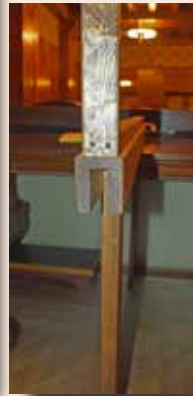
Below, the partitions are supported by one leg which provides the spacing needed for the structure to fit over the existing workspace dividers on the bench. Right, the structure is clamped onto the molding for stability.
