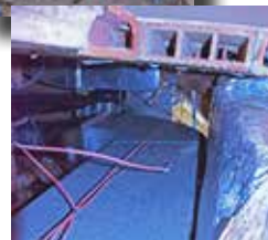
Above, looking down from the second floor chase opened in the project, above right, ducts originating in the basement come up through the first floor to enter the chase and then extend on up to the third floor where light shines, right, in the center of the image.
