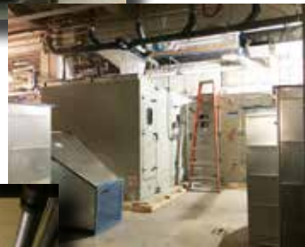
Above and left, contractors unload and move air handling units weighing up to 2000 lbs. into basement machine rooms for integration into the ventilation system.
