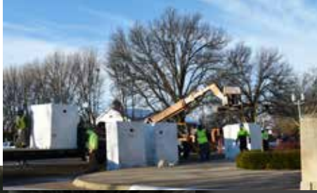
Above and left, contractors unload and move air handling units weighing up to 2000 lbs. into basement machine rooms for integration into the ventilation system.
