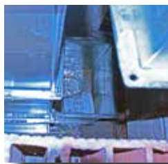
Above, looking down from the second floor chase opened in the project, above right, ducts originating in the basement come up through the first floor to enter the chase and then extend on up to the third floor where light shines, right, in the center of the image.
