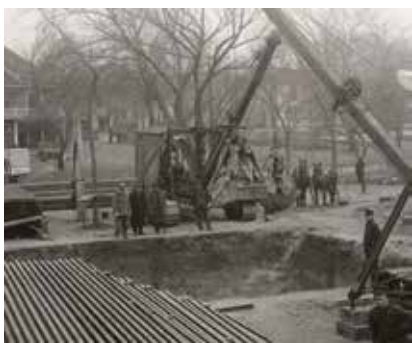
Digging the test pit on the east lawn of the 2nd Capitol took a combination of man, steam and horse power. Stacks of rails were stored on site for the test.
