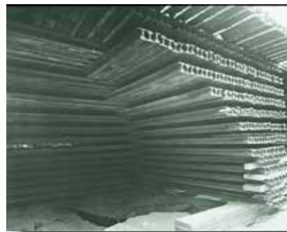
The 30 foot long steel rails weighing 560 pounds each were stacked one at a time and balanced on the punch until the stone fractured.
