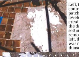
Left, the contractors patched and leveled the holes created when the damaged setting bed was removed. Below left, the loose tile was reset with a thinset mortar.
