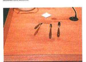
Above, after inspection staff found tears in the veneer and right, repaired and reglued the veneer in place.
