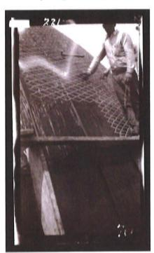
Below, detail of the dome and sprayed gunite. The concrete gunite was scored while wet to provide grip for the setting bed layer.
