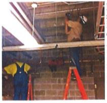
Left, in the final step of the pump installation, OCC's electrician, Tahir Karimi, hooked up the electrical power to run the pump while the plumber, Gillett, made the final connection.
