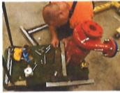
Above left, custom mounting brackets were fabricated in the shop. Above right, OCC's plumber fits the mounts to the new pump prior to mounting the pump on the wall. Right, once mounted the plumber added copper pipes to connect the pump to the exterior irrigation system.
