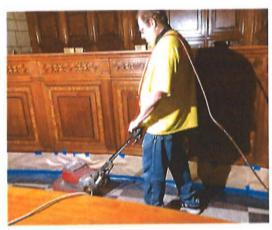
Left, after protecting the base of the judges' bench, the Richard Mallam, custodial leader, was able to use power equipment to strip the floor finish, rather than using a more time consuming hand-stripping process.
