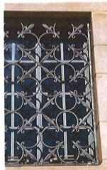
Left, the window and grille before repairs. The steel window had rusted and would not close tightly. The exterior grille finish was faded and the grille loose in the enclosure. Right, the repaired window, repainted, reglazed and operational. The repatinated grille matches the window color and is securely installed.
