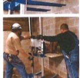
efficiency. In the mid-1990's a concrete block wall was installed to provide additional shop and storage space in the basement. This new wall allowed Gillett an alternate way to mount the pump.
