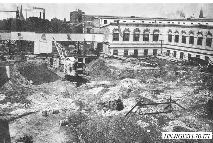
By August 1, 2025, all that remains of the second Capitol is scattered rubble. Excavation of the footings, foundation and basement will be done from within the outer square. A rail line will be brought into the center under the east and west walkways. Excavation cranes will place the removed soil into railcars to be carried away and used for fill at the State Fair, now Innovation Campus, site along Salt Creek.
