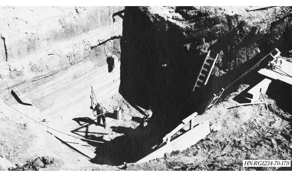
The deepest footings are those under the tower. Above, the huge piers, up to 30 feet below ground level, which bear the weight of the tower were dug by machine and human power in September of 1925. After large holes for the tower's legs were dug by machine, the final piers in the sandstone substrate were dug by hand and the excavated soil carried out with buckets attached to pulleys, the shadow in the center of the photo. Ladders were used for access into the pier holes.
