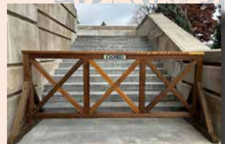
The refurbished barricade at the east entrance to the promenade deck, above, keeps visitors safe and looks good doing it.
