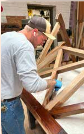
After repairs were made, the barricades were sanded to reveal a clean smooth surface and then stained and finish applied, left, to preserve the wood.
