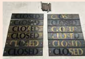
In addition to refurbishing the barricades, staff worked to improve the finish on the 'CLOSED' signs. Right, the paint on the signs was damaged and the finish was uneven.
